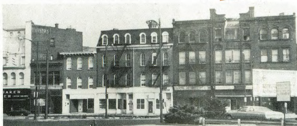
Southeast side of Genesee Street Between Ellicott and Oak
