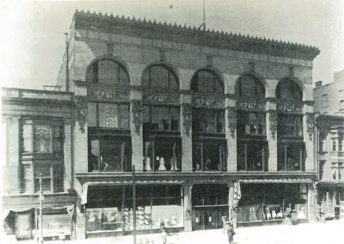
Flint and Kent building - before "modernization"
