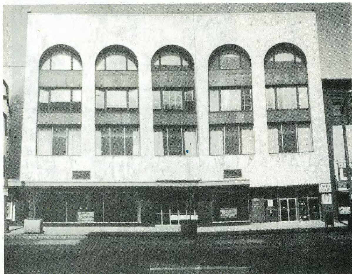
Flint and Kent building - after "modernization"
