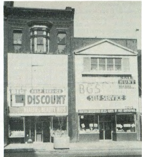
West side of Main Street 500 block
