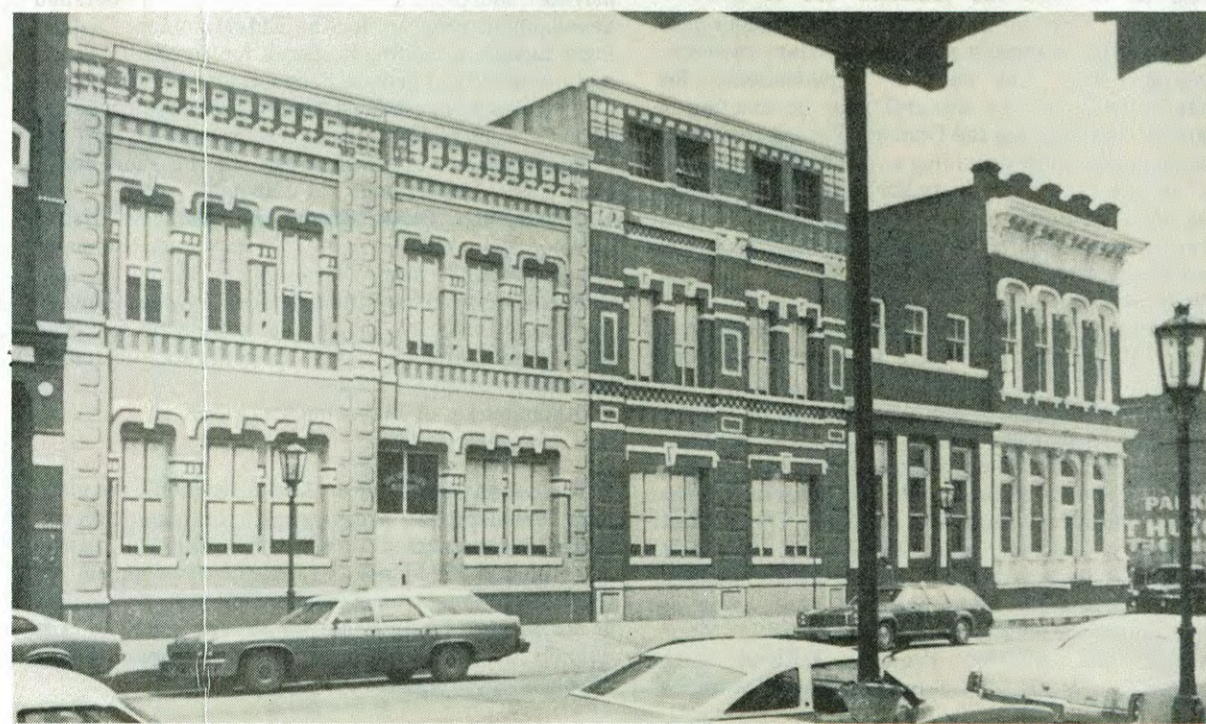
Trompe L'Oeil facades in the Strand, Galveston, Texas Painted in 1976 to suggest missing cast iron decoration. (left to right: painted, painted, and real)
