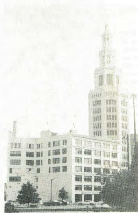
Niagara Mohawk Power Company Tower From the north
