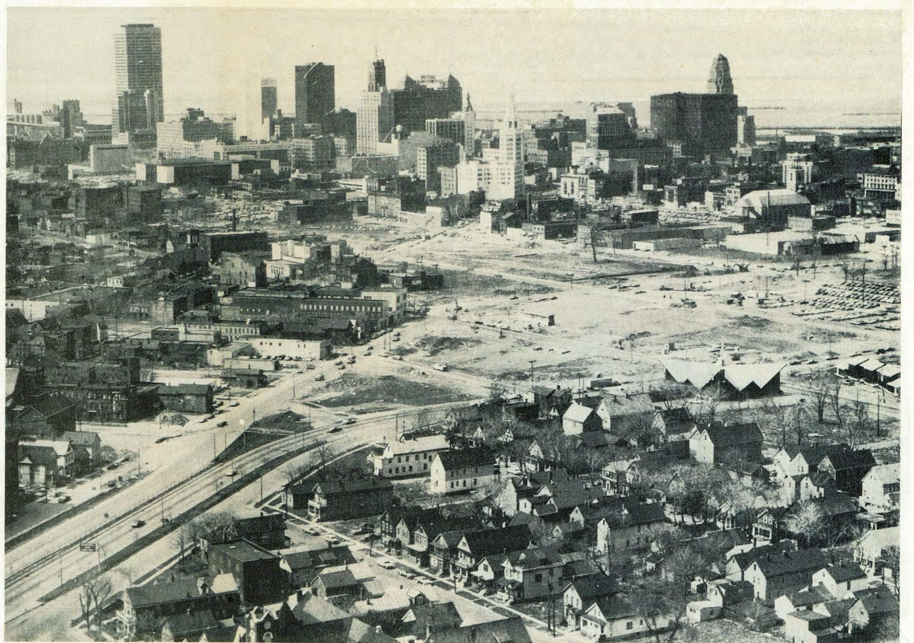
Downtown Buffalo from the north east Showing Kensington Expressway and cleared site for Elm-Oak Arterial in foreground with Central Business District top left and Entertainment District top right.
