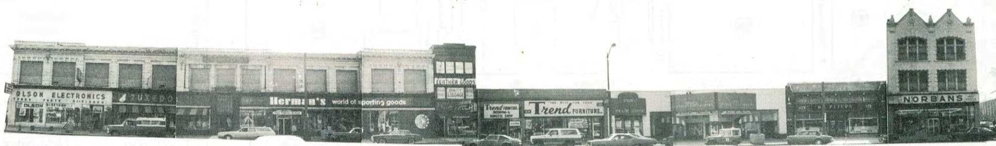
East Side of Main Street 600 Block - north end
